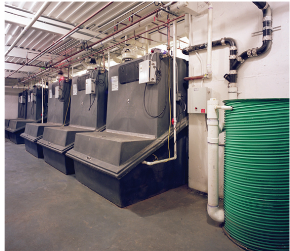
Composting equipment in the basement of the Eco-Restroom holds waste as it composts into stable fertilizer.
